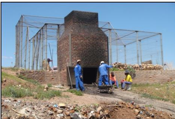
Figure 10: Incinerator used on site to burn waste
