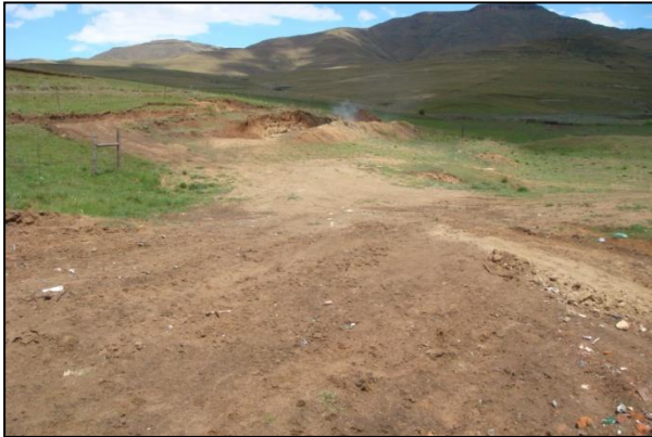
Figure 14: Overview of Rhodes Landfill Site
