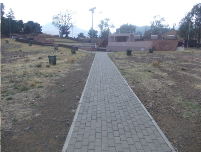
Image 50: Brick Paving in Barkly East
