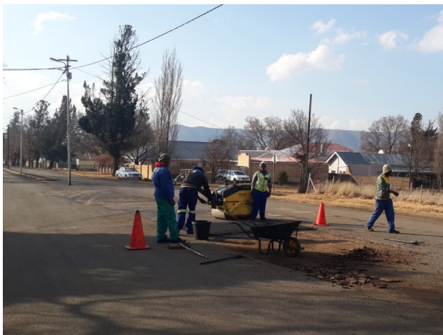
Image 43: Road Maintenance in Lady Grey
