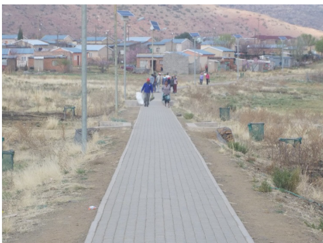
Image 49: Brick Paving in Barkly East
