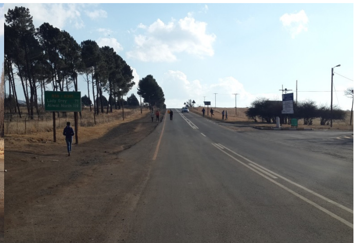
Image 44: Lack of Paving in Barkly East
