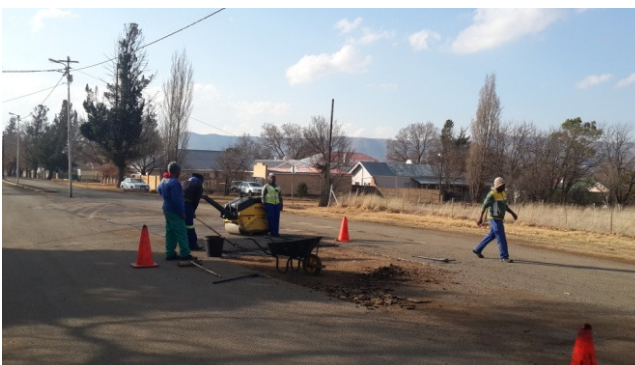
Image 41: Road Maintenance in Lady Grey
